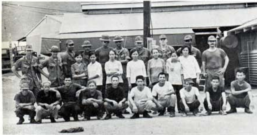
Keep the mess hall operating
