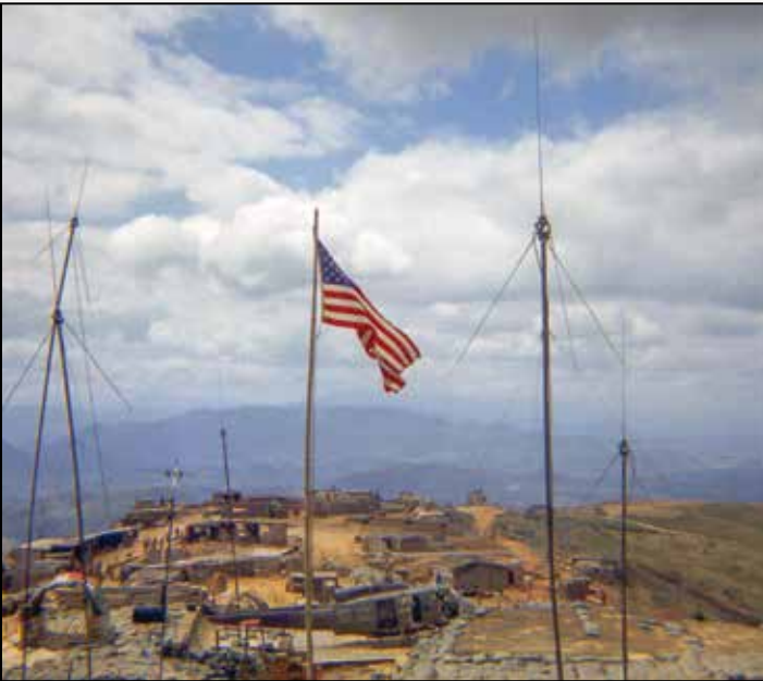
Slick on VIP pad. BTOC under sandbags. 292 antennas for my radios.
